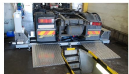
BM20200 installed in existing pit
